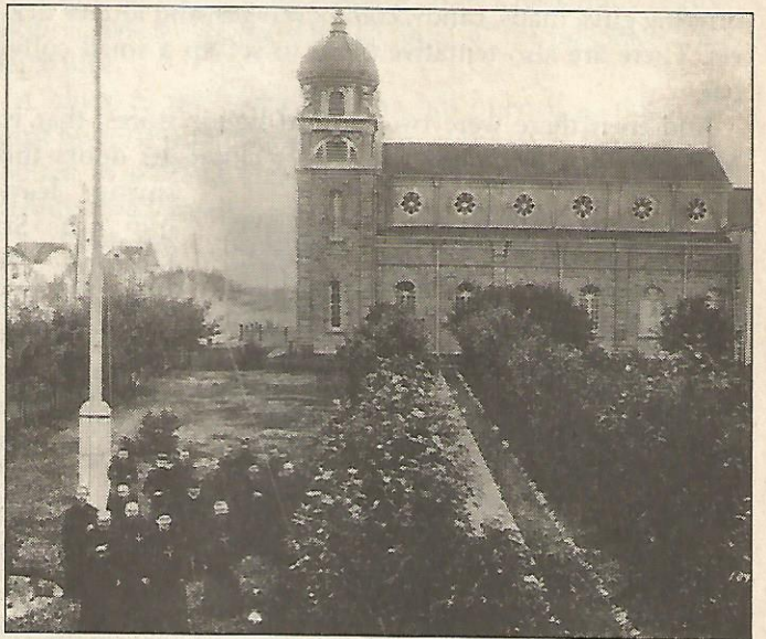
EARLY TRANSFORMATION: Calgary's first Catholic mission was erected on bald prairie in 1883 (top); Trees and shrubs had transformed the landscape by 1910.
