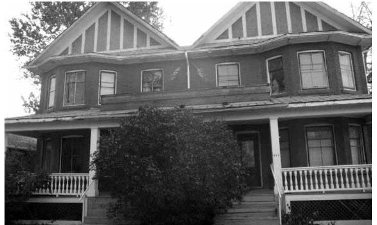
SOMERVILLE DUPLEX PHOTO BY KIM MUNCHRATH
